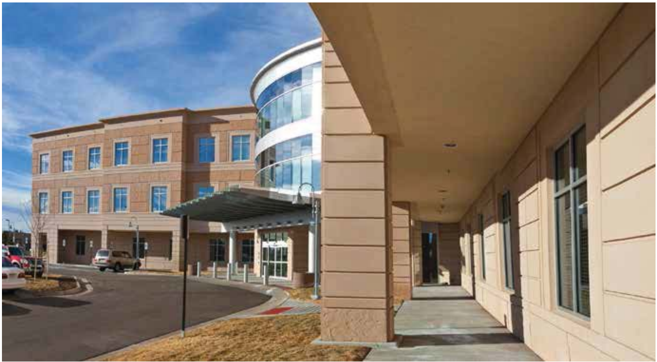
The two-story, upper-level panels feature a darker color in a flagstone texture, while the first floor used a buff-colored limestone look with wide reveals. The rectangular pattern continued onto all four sides of column covers on the entry colonnade. Photo: Rocky Mountain Prestress.
