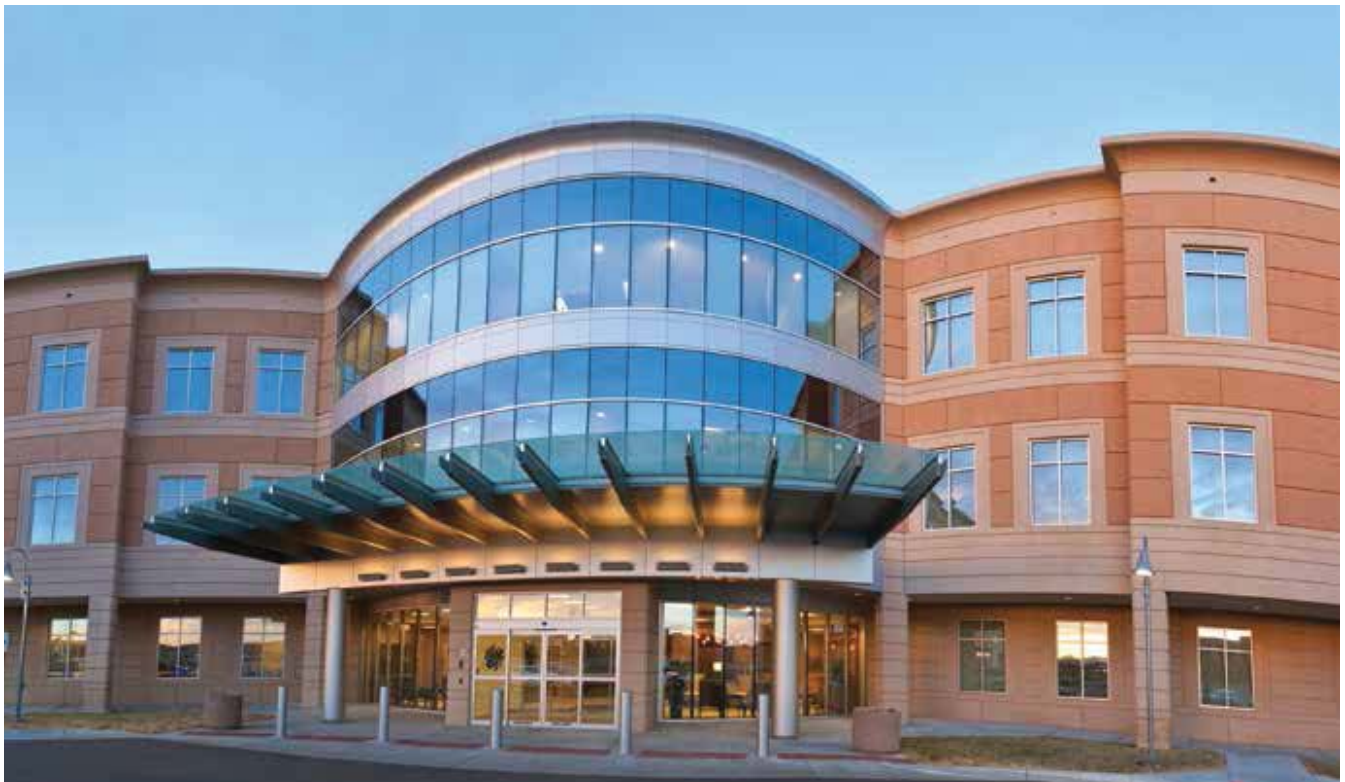
When the original steel and masonry design for The Center at Lincoln, a skilled nursing facility in Parker, Colo., proved economically unviable, a total precast concrete system was used. It consisted of 64-foot-long double tees, columns, beams, and load-bearing architectural wall panels. Photo: Rocky Mountain Prestress.
