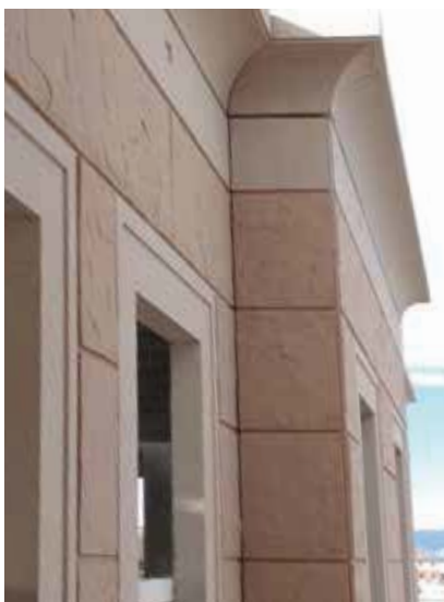
A curved cornice was added to the panels on the top floor, creating a distinctive roofline. Photo: FDG Inc.
