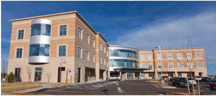
Two-story bay windows reflect the rounded curtain wall used at the entry. The windows rest on a curved precast concrete slab that cantilevers off the wall panels. Photo: Rocky Mountain Prestress.
